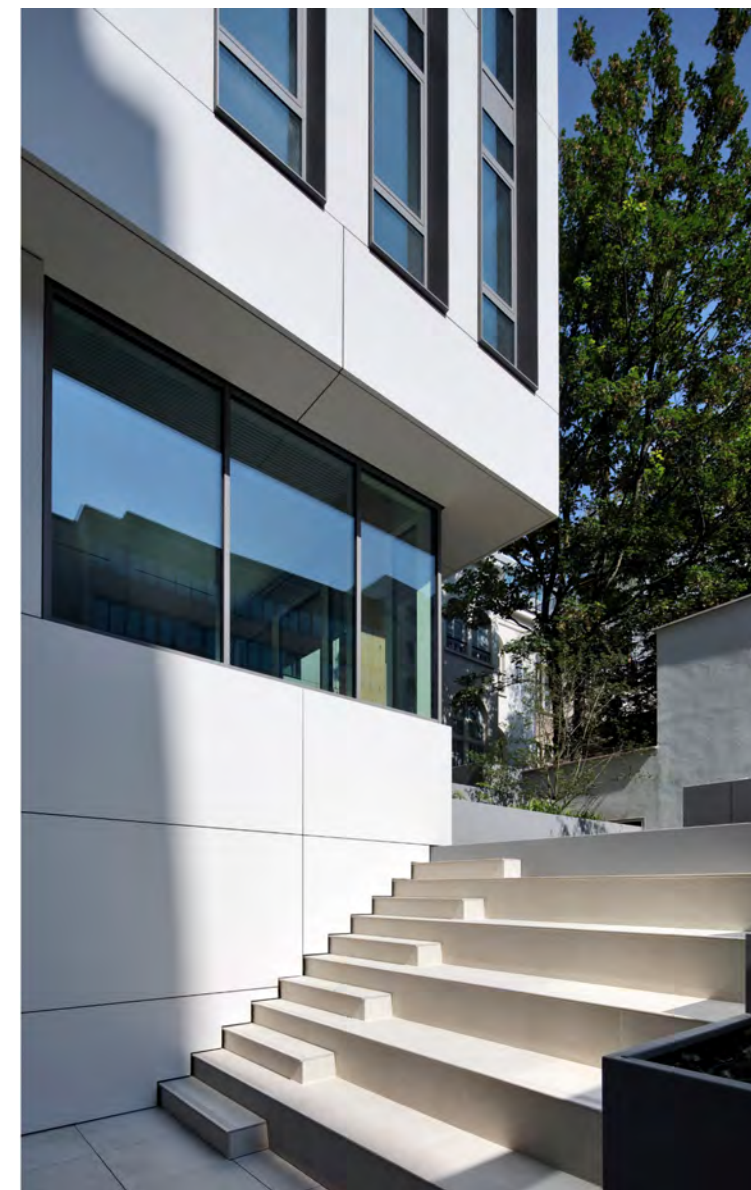
► Office building Montoyer 10 (M10) - Brussels' CBD (BE)
